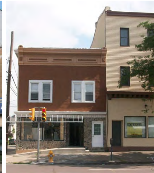
Example where a building undergoing renovation has been painted with colors compatible with the adjacent building. Complimentary stone veneer has been added to the ground floor façade and the existing cornice have been painted to accentuate its detailed molding. Source: Barry Isett & Associates, Inc.
