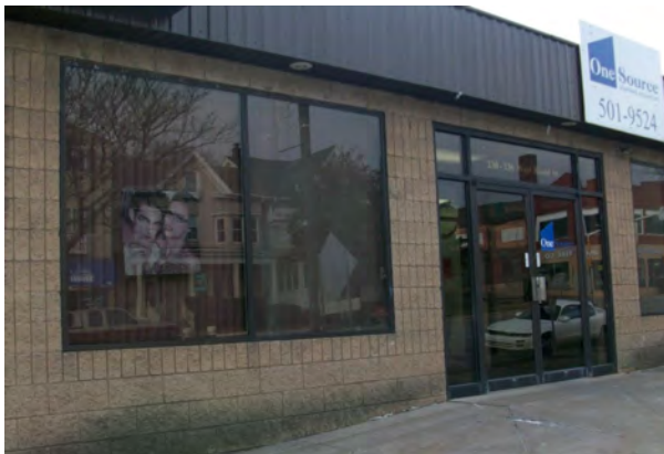
Reflective, black glass and glass tinted more than 40% in windows and doors is prohibited on the ground floor facade. Source: Barry Isett & Associates, Inc.
