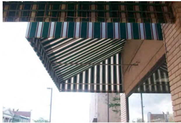
Example of canvas awning affixed to the Broad Street Business Exchange. Source: Barry Isett & Associates, Inc.
