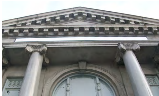
Example of how the ca. 1924 American Bank and Trust Company (deemed eligible for listing on the National Register) has distinct Neoclassical architectural features that should be preserved, including the portico, stone columns, and decorative cornice. Source: Barry Isett & Associates, Inc.
