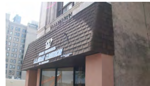
Example where a building undergoing renovation has been painted with colors compatible with the adjacent building. Complimentary stone veneer has been added to the ground floor façade and the existing cornice have been painted to accentuate its detailed molding. Source: Barry Isett & Associates, Inc.
