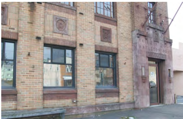
Example of how the 1928 American Legion Building (deemed eligible for listing on the National Register) has distinct Art Deco architectural features that should be preserved, including the pane windows, stone window sills, stone carvings, unique brick patterns and colors, and projecting entry. Source: Barry Isett & Associates, Inc.
