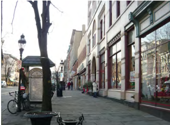
Example of how a consistent build-to line and buildings with large windows at street level create a comfortable and interesting pedestrian environment (Bethlehem, PA). Source: Barry Isett & Associates, Inc.
