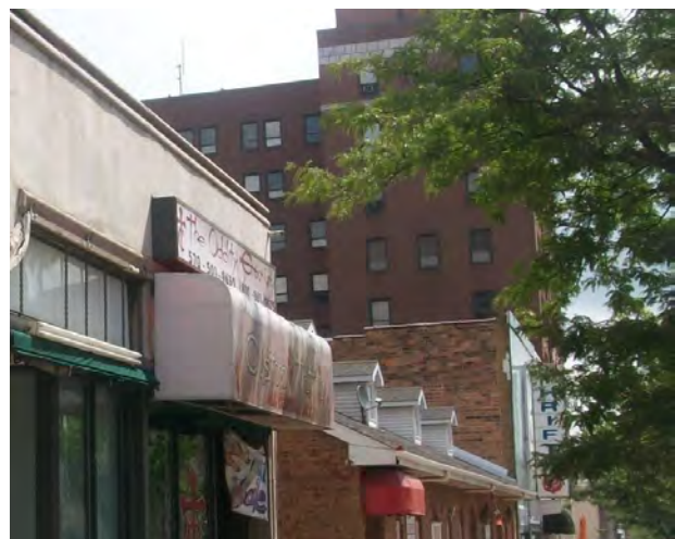
Two examples of awnings that do not meet the standards of this ordinance. In both cases, the awnings are too narrow and constructed of plastic. In the example at left, the amount of text also makes it appear cluttered, and an awning constructed as part of the building already exists above it, so it appears awkwardly placed. In the example at right, the awning obscures the transom window above the storefront and detracts from the character of the building. The example at left also has too many signs affixed to the building façade, as no commercial establishment shall be permitted a total of more than two signs. Source: Barry Isett & Associates, Inc.
