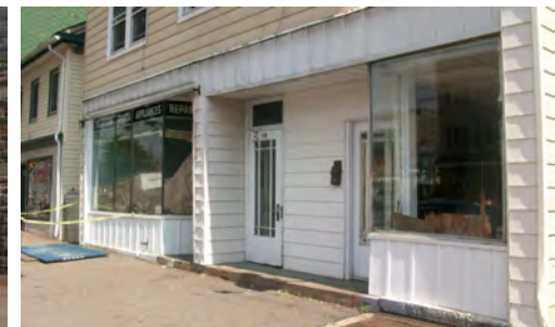
Asphalt shingles and aluminum siding are not permitted on building facades at the ground floor level. Source: Barry Isett & Associates, Inc.
