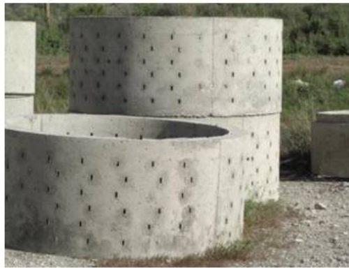
Figure E.4. Dry Well #1 – Structural Prefabricated Chamber.
